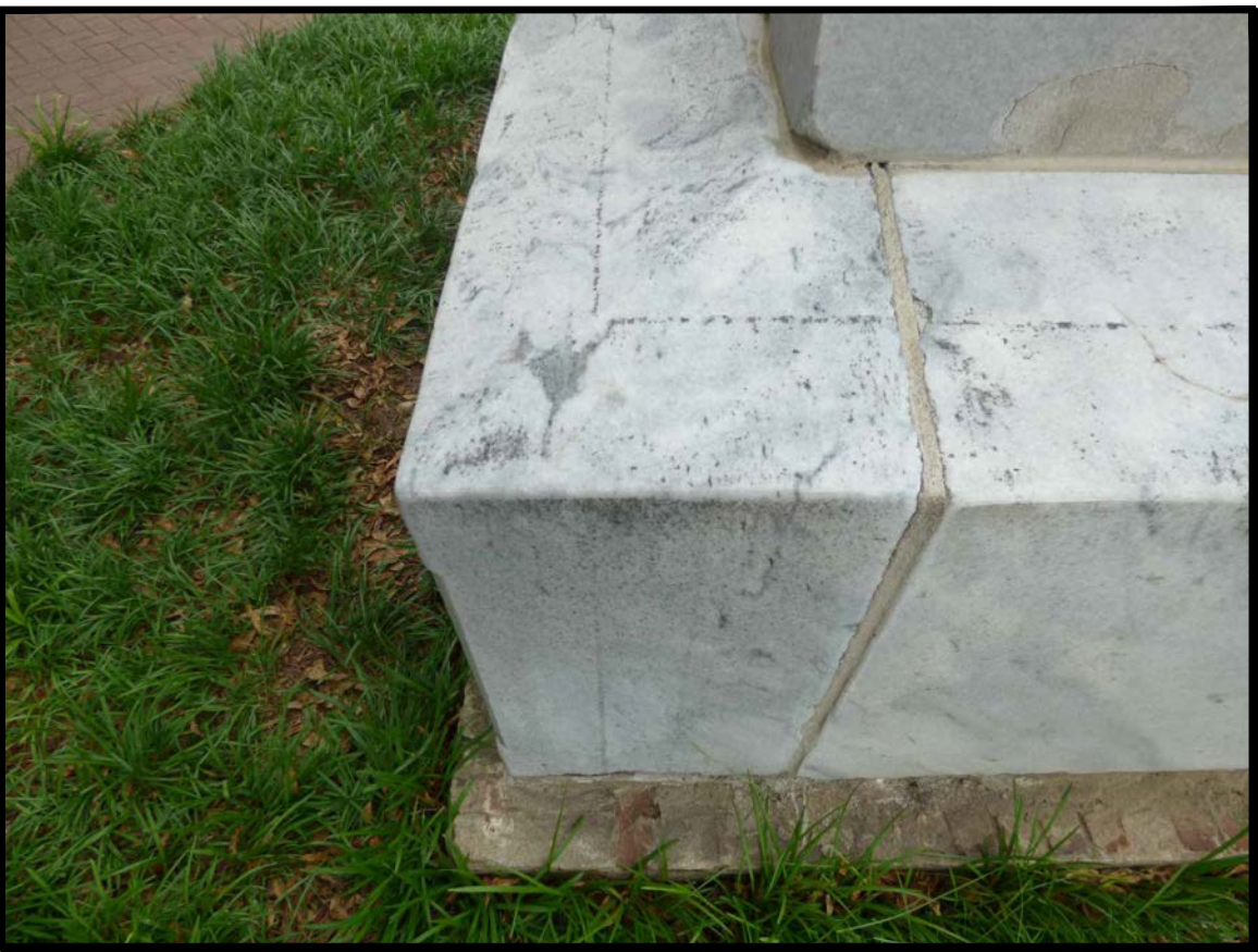
TYPICAL VERTICAL JOINT at 4 PIECE BASE
